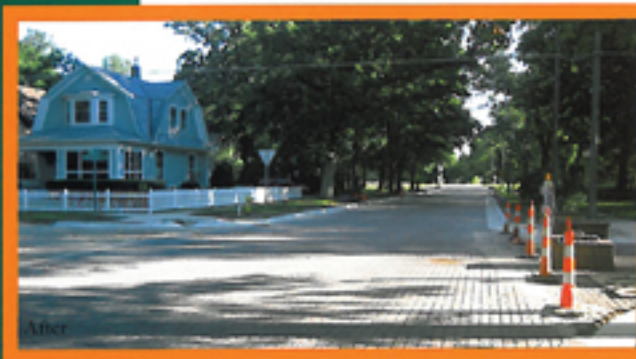
A neighborhood in Charles City suffered from poor roads and storm water drainage problems before the city installed permeable pavers.
