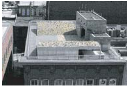
green roof view from adjacent building
